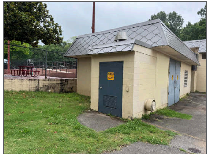
Chemical Storage Entrance
